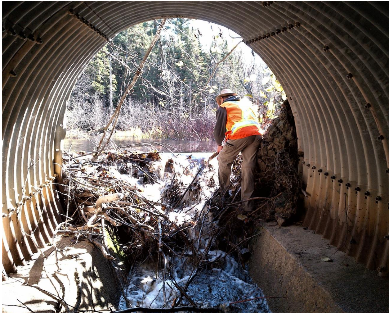
Figure 11 Notching a Beaver Dam to Allow Fish Passage
